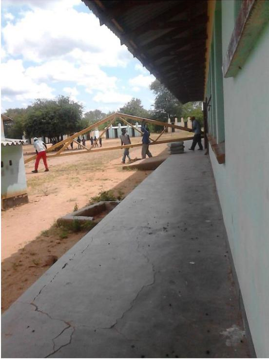
The roof truss was put together at the school. Here is the first part on its way to the new block.
