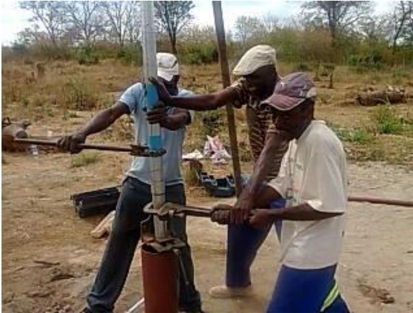
The next step: A thinner pipe is screwed together, piece by piece, until it has reached a depth of 60 metres. It is through this second pipe that the water will be extracted.
