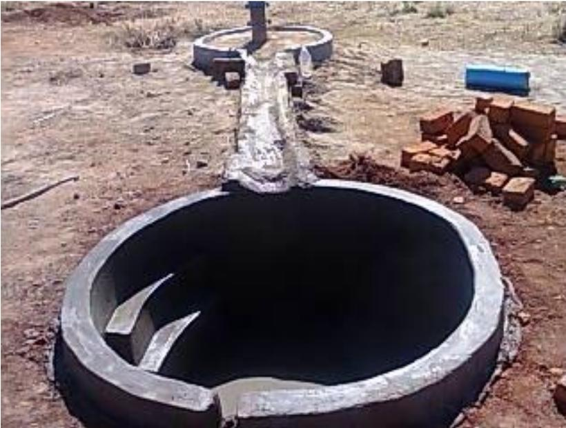
The well can be seen in the background, with the channel leading to the first catch basin in the foreground. PVC pipes distribute the water from here to tanks in the school garden.
