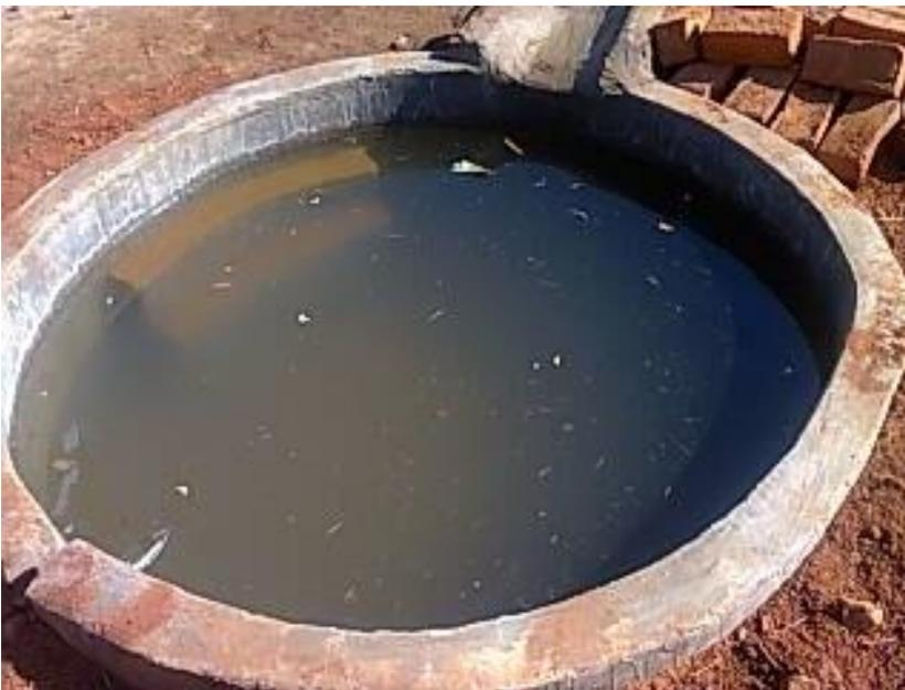
The first catch basin has passed its seven-day test - it is watertight!
