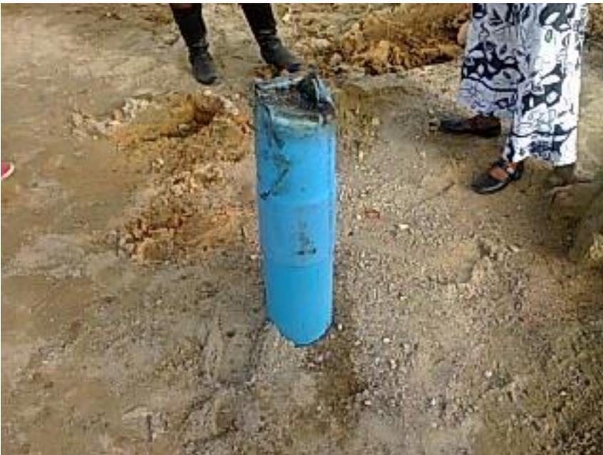
The drilling work is finished. All that is visible at this stage is the end of the 60-metre drill pipe, covered by a protective cap.
